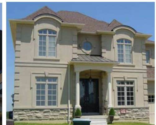
Figure 6.3.5f - Example of Stucco-Clad Dwelling
