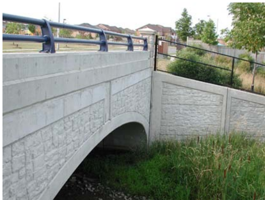
Figure 5.8c - Intended character of Bridge design, end pier, and box beam guide rail
