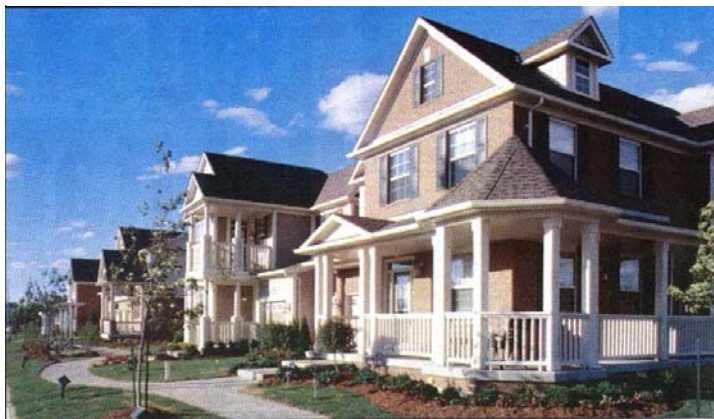
Figure 3.2a - All Publicly Exposed Façades Shall Exhibit a High Degree of Design Quality
