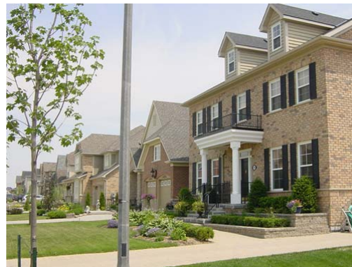
Figure 2.2a - A Well-Defined Street Edge Contributes to the Pedestrian-Oriented Goals of the Community
