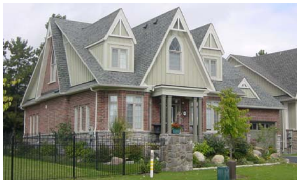
Figure 6.3.5f - Example of Dwelling with Fibre-Cement Siding / Wood Siding as an Accent Wall Cladding Material
