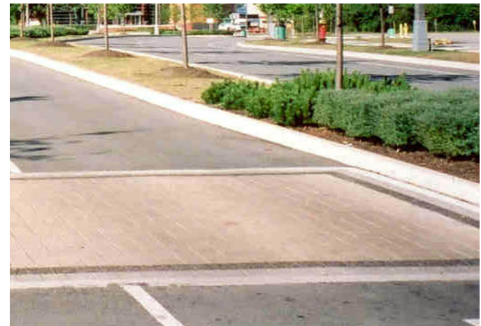
Figure 4.2v - Coloured concrete at crosswalks
