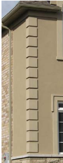
Fig. 6.3.13b - Correct Application of Stucco Quoining (Even Spacing)
