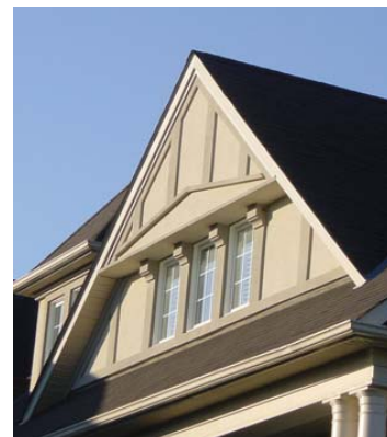
Figure 6.3.5e - Example of Stucco Detailing
