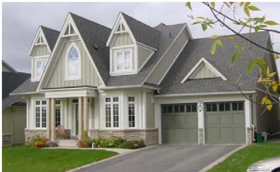
Figure 6.3.5e - Example of Dwelling with Fibre-Cement Siding / Wood Siding as a Main Wall Cladding Material
